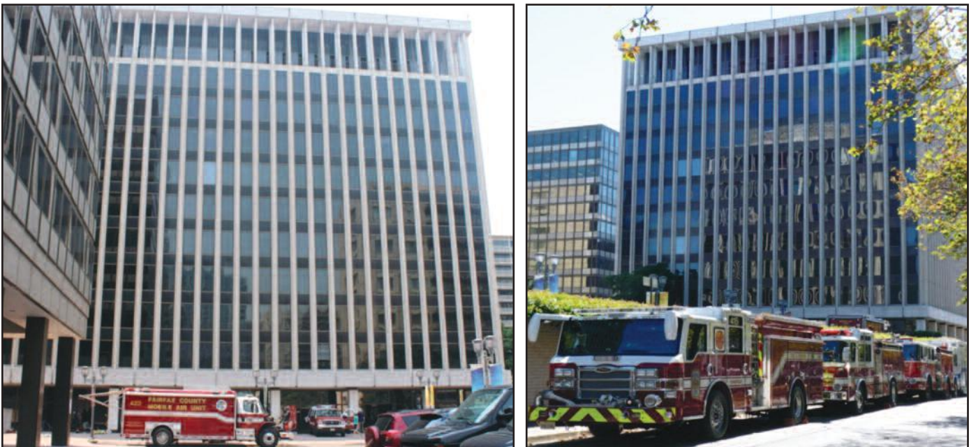
Figure 1: High-rise building located at 223 23rd Street, Crystal City, VA
