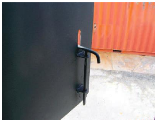
Figure C-6: Window & Latch Construction
