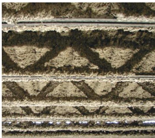
Figure C-4: Fireproofing added to structural steel
